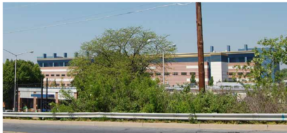
Forest Glen Annex Research Facility
