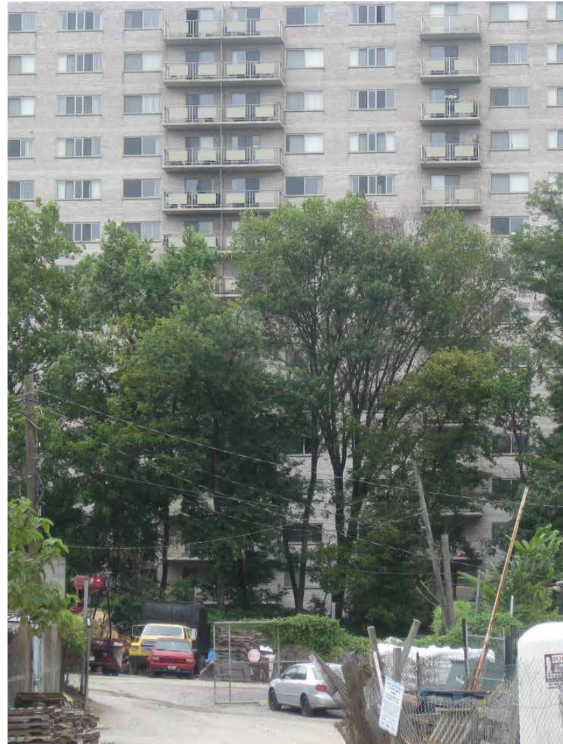
Inadequate buffering between residential and industrial land uses
