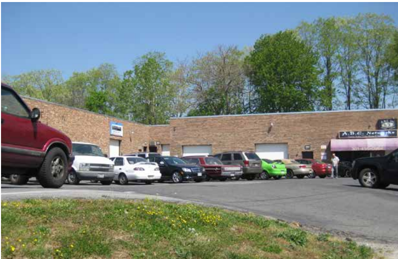
Opportunities exist for façade improvements to industrial buildings
